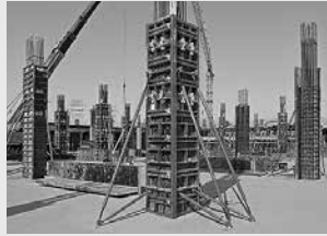
Column Formwork
