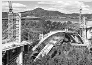
Bridge Formwork
