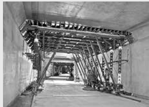
Tunnel Formwork
