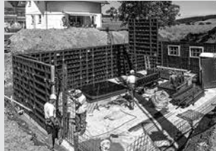
Wall Formwork
