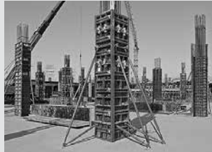
Column Formwork
