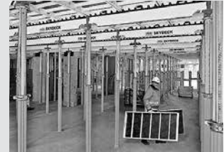
Slab Formwork
