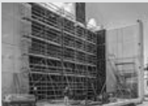
Working scaffolds construction
