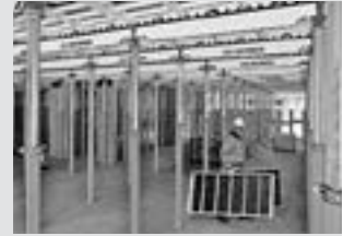
Slab formwork
