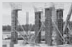
Column Formwork
