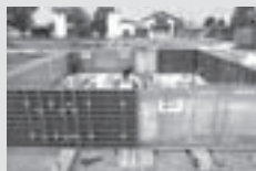
Wall Formwork
