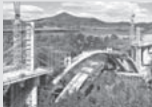
Bridge Formwork
