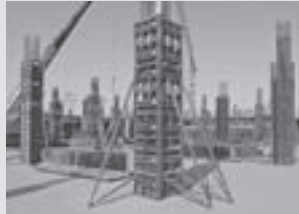
Column Formwork
