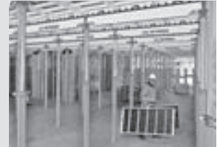
Slab Formwork
