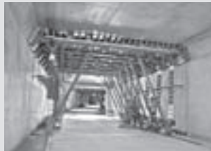
Tunnel Formwork
