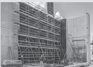
Working scaffold construction
