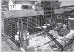
Wall formwork
