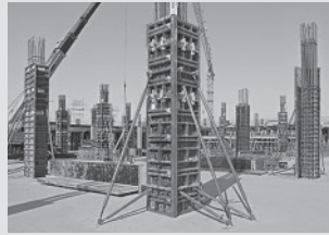
Column formwork
