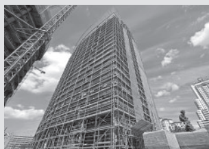
Working scaffold façade
