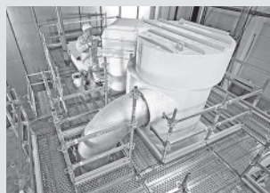
Working scaffold industry
