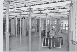
Slab formwork
