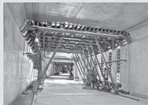
Tunnel formwork
