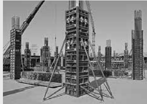
Column Formwork
