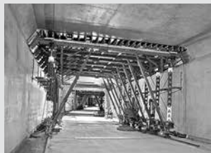
Tunnel Formwork
