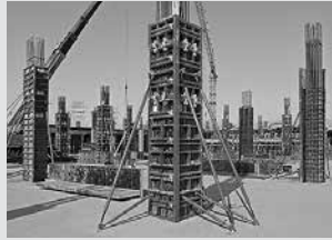
Column Formwork
