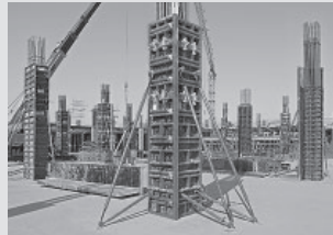
Column formwork
