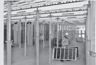
Slab formwork
