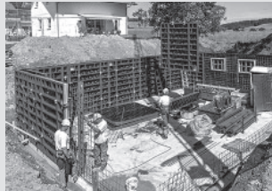
Wall formwork
