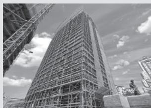
Working scaffolds facade
