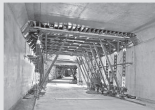
Tunnel formwork
