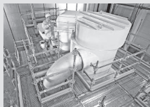
Working scaffolds industry
