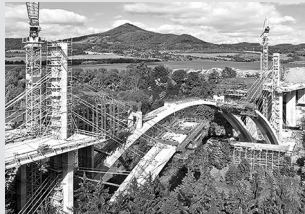
Bridge formwork
