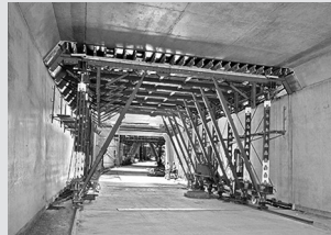
Tunnel formwork
