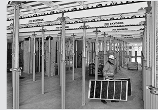
Slab formwork
