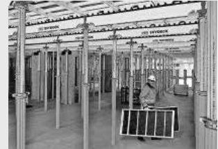
Slab Formwork
