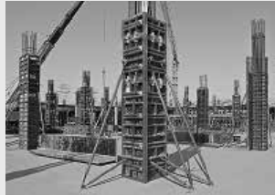
Column Formwork
