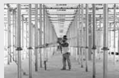
Slab Formwork
