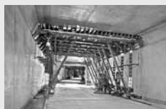
Tunnel Formwork
