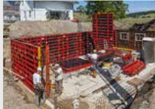
Wall Formwork
