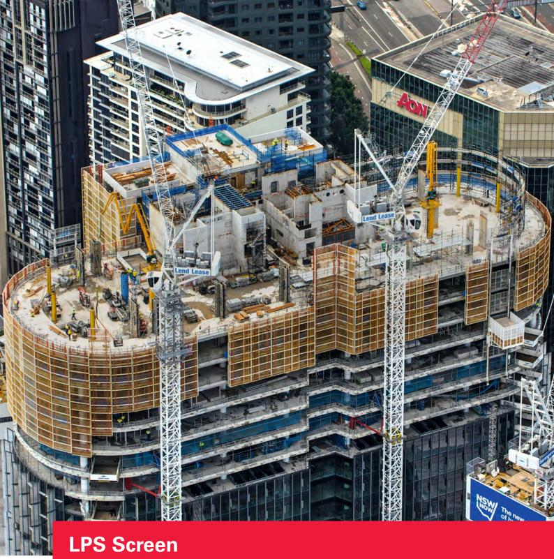
The lightweight climbing protection panel with mesh enclosure
