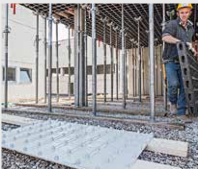
3. Installing the new formlining
