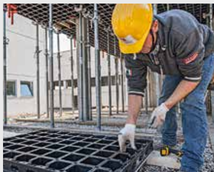
4. Screwing on the new formlining
